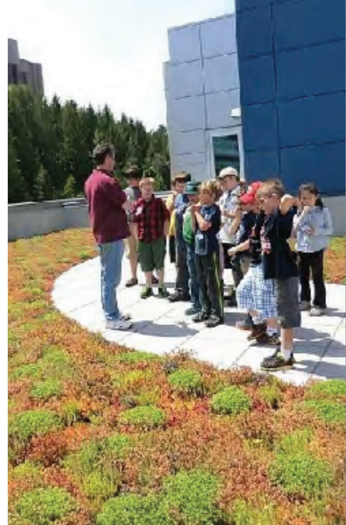
A carpet of plants on many of the second-floor roofs at the GLRC soak up runoff and act as natural temperature regulators—helping to keep the building cool in the summer months.
